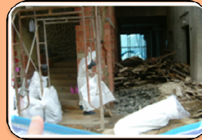
Removal of asbestos
