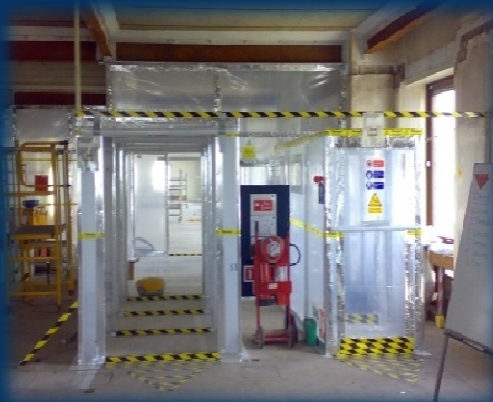
Designated work area
